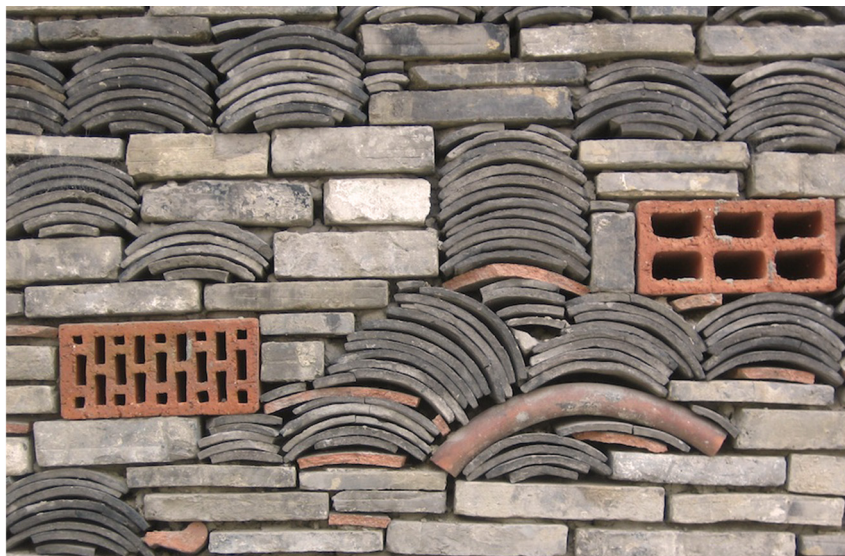
Fig. 8 Detail of the wall pattern. Materials assembled using the ‘wapan’ technique.
