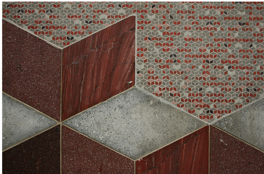
Fig. 6 Detail of the wall pattern: a riot of coloured stonework – quartzite, porphyries and Ancaster limestone.
