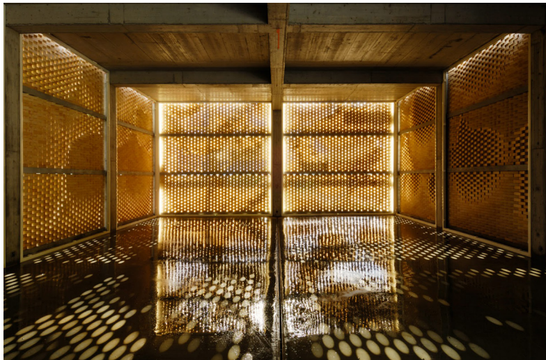
Fig. 13 Interior of the vineyard. The masonry pattern at the same time filters and allows the light coming in.
