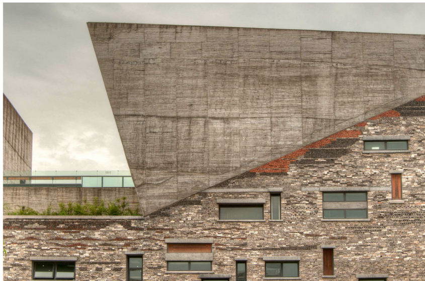
Fig. 7 The south elevation of the museum shows the relationship between the concrete part of the facade and the one made by debris.
